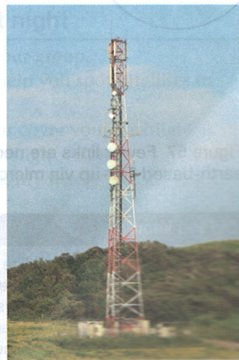
Figure 55 A microwave tower with dish antennas
