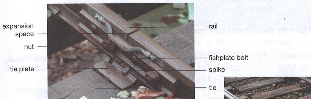
Figure 48 Fish plates are used on railway tracks to join sections of railway track and allow for expansion due to heating.
